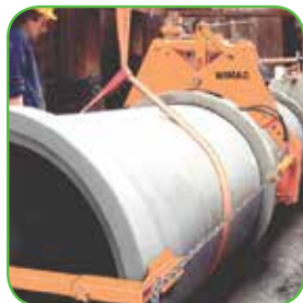
Pipe Pulling Device
