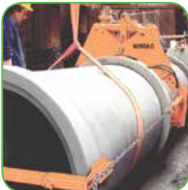
Pipe Pulling Device
