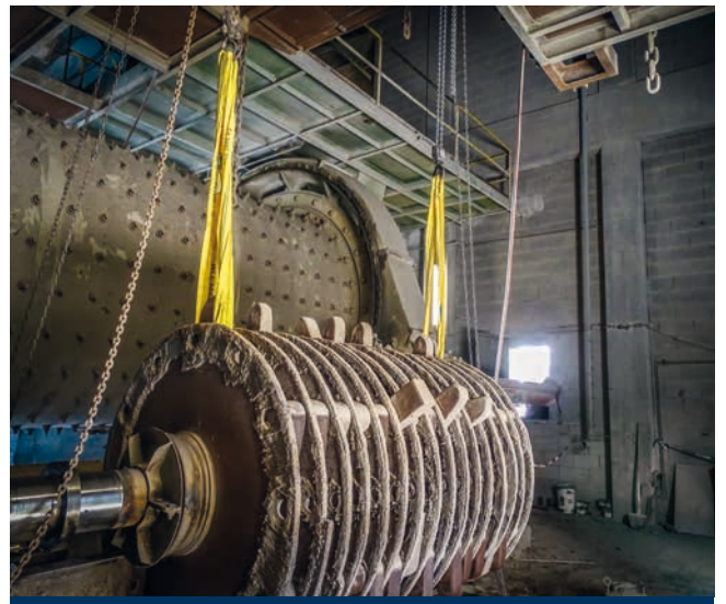
Lifting operation using round slings
